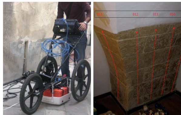
Figure 14. Ground penetrating radar scan: foundation line; vault.
