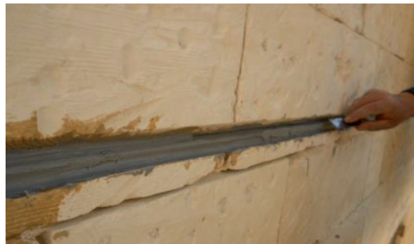
Figure 20. Application of the CFRP pre-tensioned wires.
