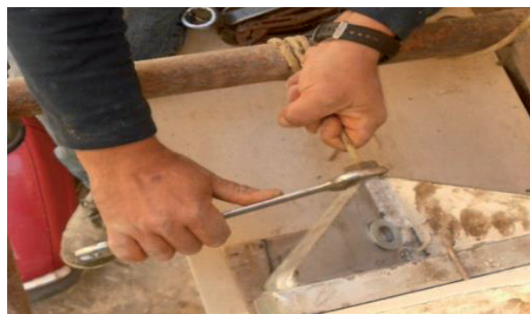
Figure 20. Application of the CFRP pre-tensioned wires.
