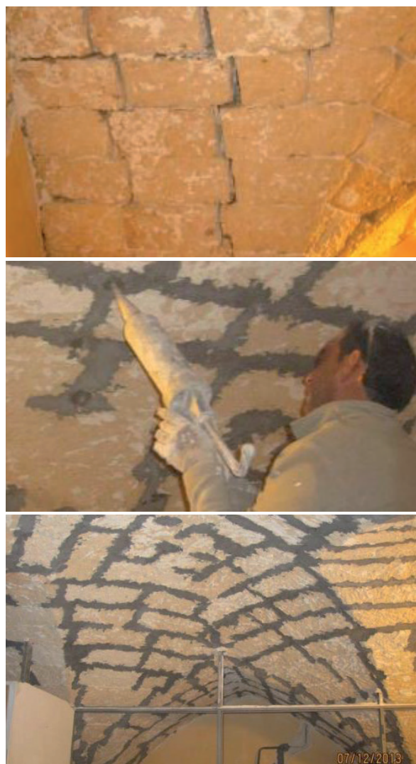
Figure 17. Injection of mortar at the vault intrados. a) before strengthening b) strengthening c) after strengthening.
