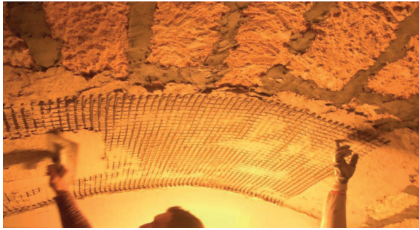
Figure 18. Installation of FRCM glass fiber system.
