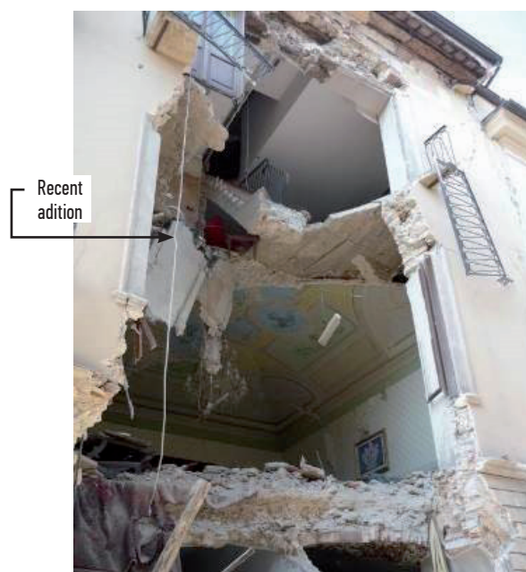
Figure 8. Damage resulting from insertion of concrete stair.
