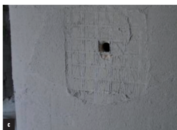
Figure 10. Application of mortar followed by carbon fabric and spikes.
