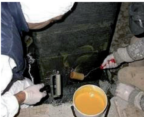
Figure 5. Strengthening of column by full CFRP wrap.
