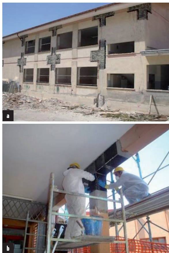
Figure 3. Prep work and strengthening of external joints.
