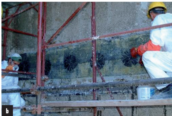
Figure 9. Wrapping with CFRP plies anchored with CFRP spikes.
